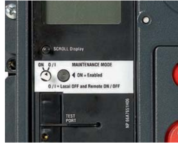
Direct ARMS activation on the circuit-breaker
