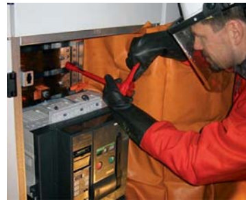
Maintenance of a switchgear system
